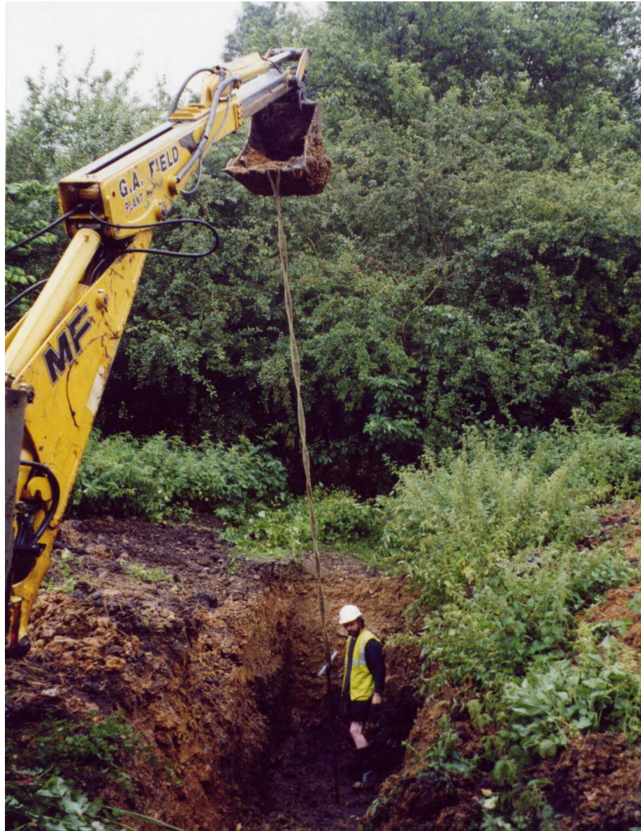
21. Obtaining soil sample by auger, with the aid of an Excavator.
